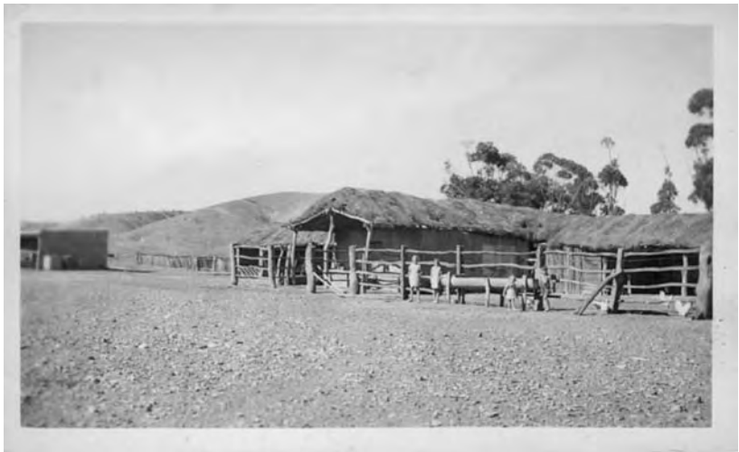
Dutton's Trough, late 1940's. Note the straw-thatched roofs on the barn and cowshed.
